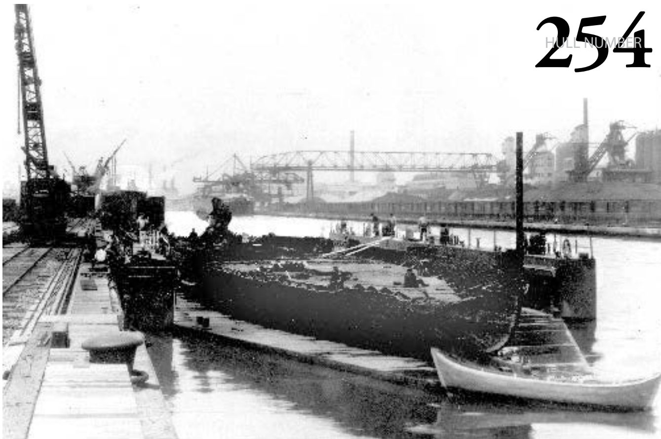
Ford dry dock showing hull remnant ("canoe") in final stage of scrapping [WG]
